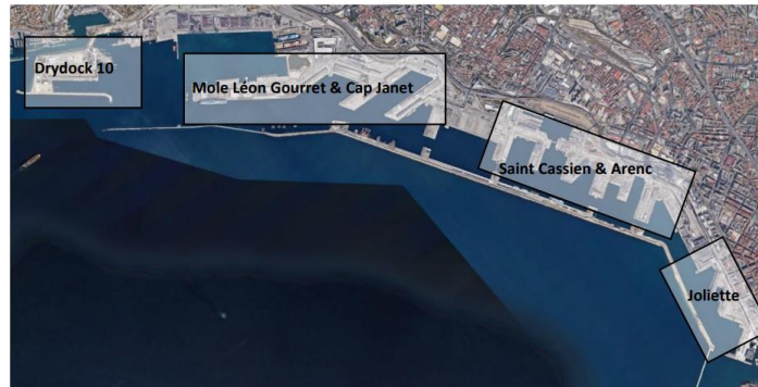
Figure 2. GPMM areas that may be available for PV panel installation.
